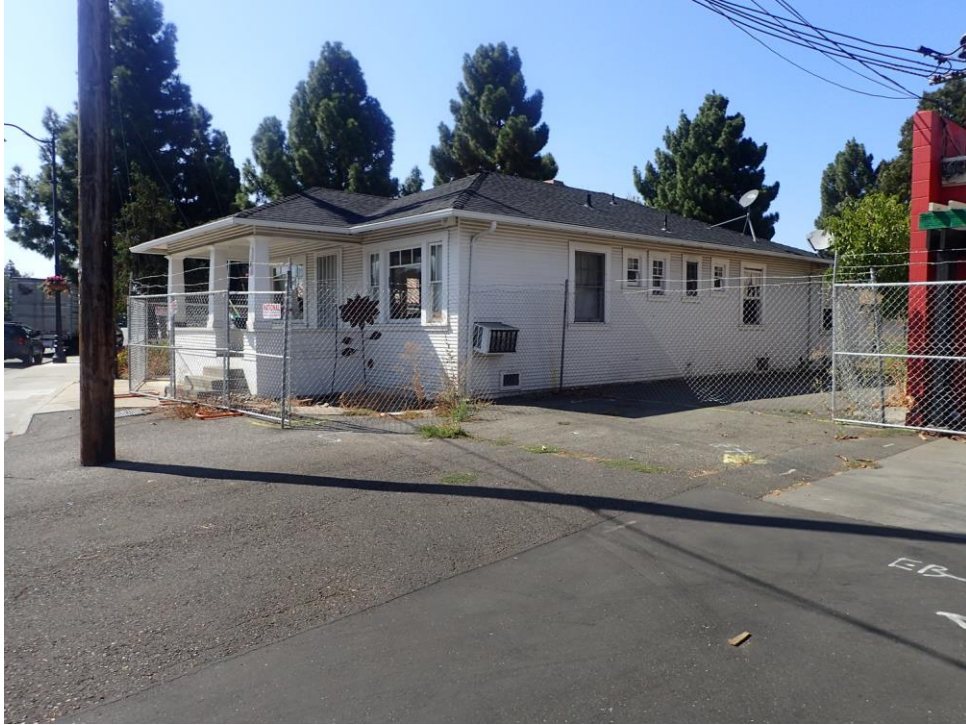
View from El Camino Real, viewed facing northwest.
