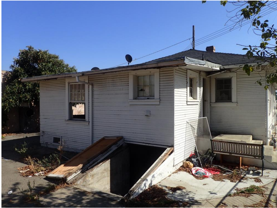
Rear elevation with shed addition, viewed facing southeast.
