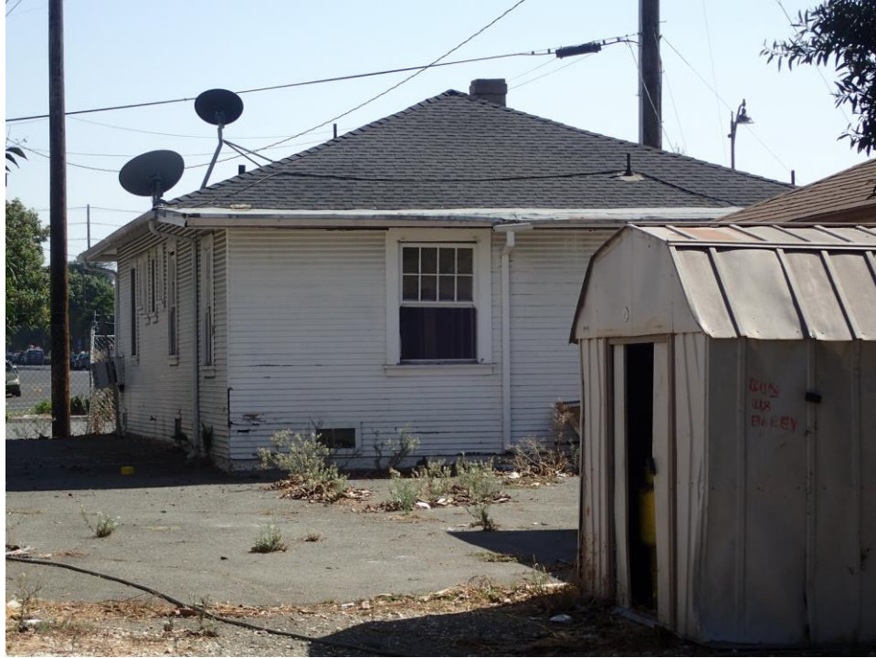
Rear shed addition viewed facing south.
