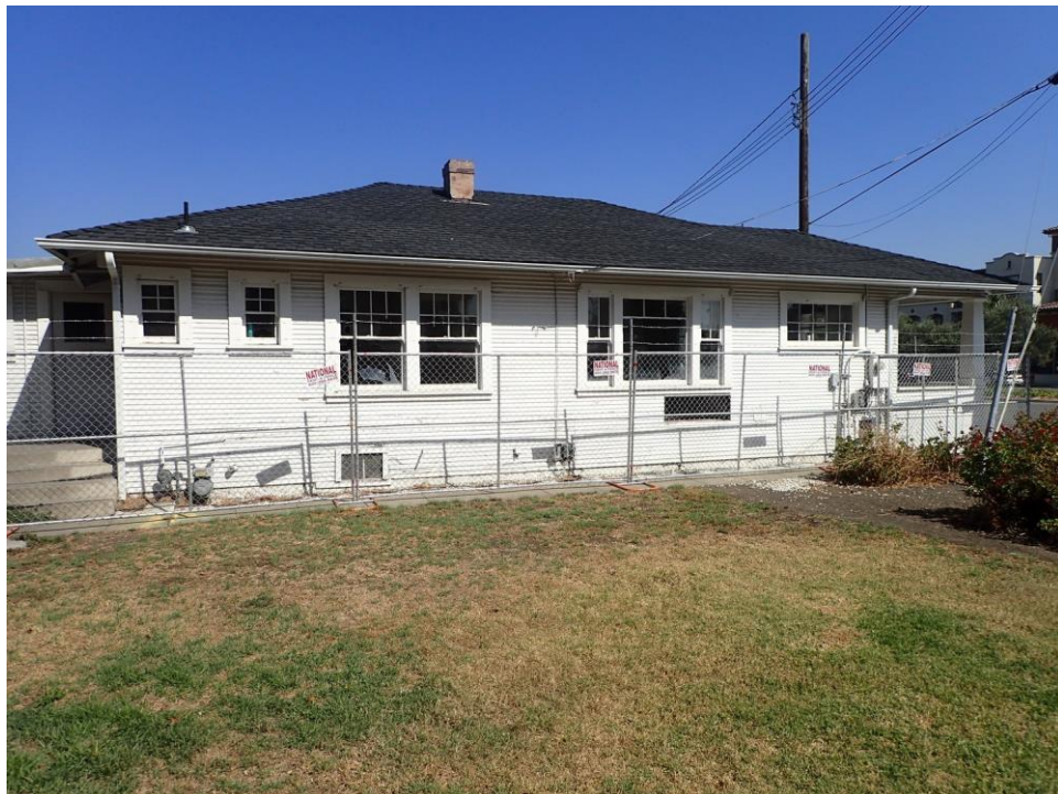
West elevation viewed facing east.
