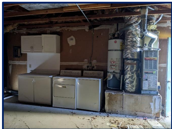
Typical interior of the garage
