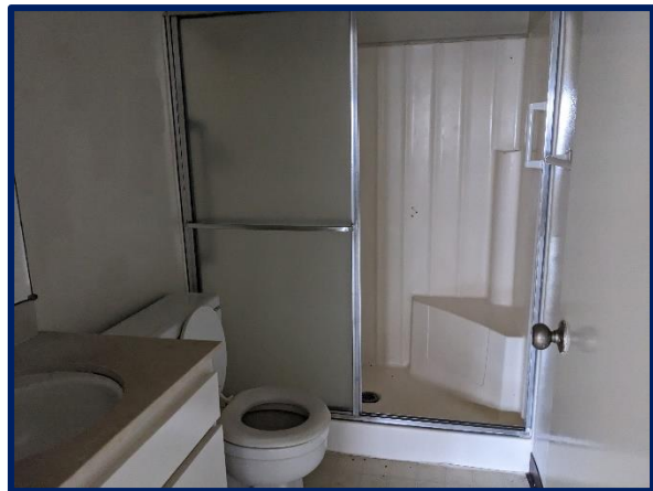
View of the property restroom
