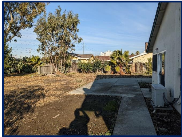
Rear of residential structure
