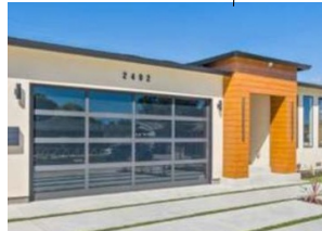
FRONT PORCH WOOD SIDING MATERIALS
