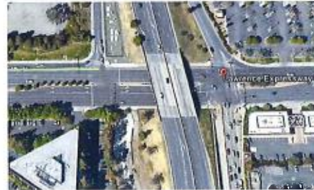
Lawrence Expressway ramp improvements
