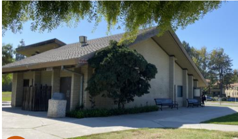
01 Community Room/ Restroom Facility
