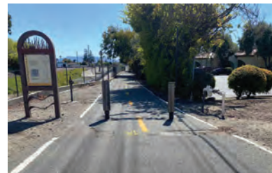
San Tomas Aquino Creek Trail Crossing.
