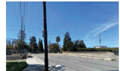
San Tomas Aquino Creek Trail Bridge von Walsh Avenue.
