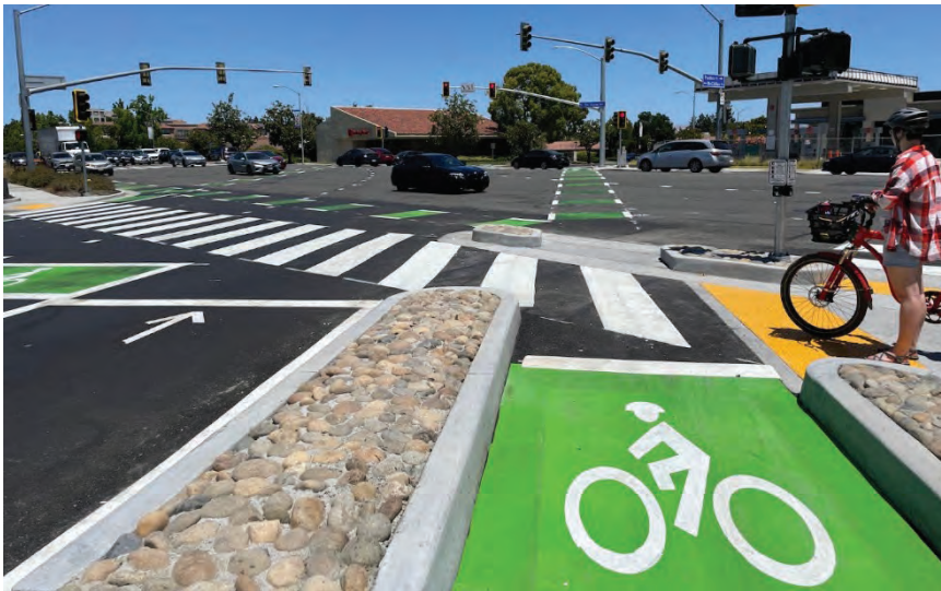
Figure 16: Protected Crossing on McClellan Road in Cupertino
