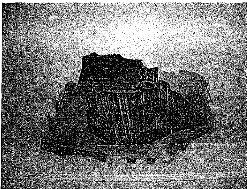
Photo 20: Detail of exposed lathe in the kitchen ceiling.
