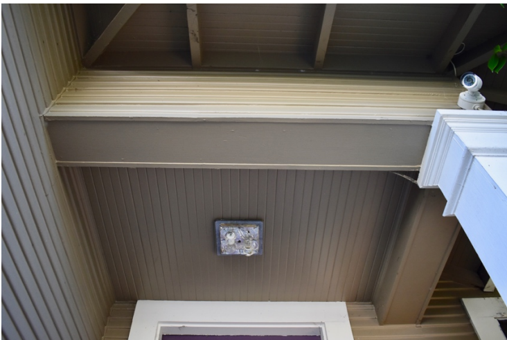
Top two photos: Front entrance, concrete porch and step, and porch post with moldings. Bottom photo: Ceiling of the recessed entrance.
