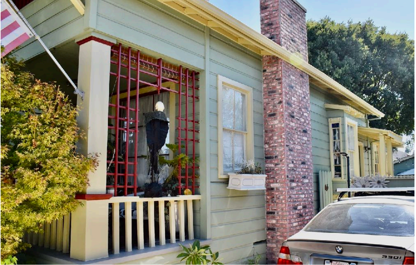
The right (west) side of the house, looking toward the rear
