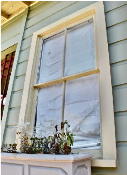
At left: Two-over-two window between main porch and chimney.
