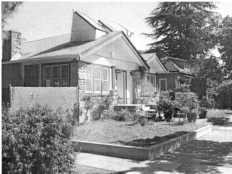
View of front façade facing east.
