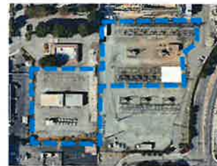
Kifer Receiving Station
