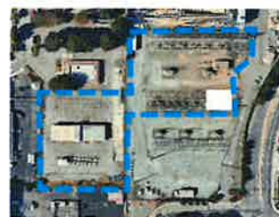
Kifer Receiving Station
