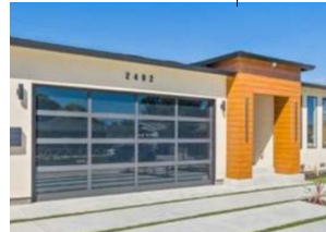
FRONT PORCH WOOD SIDING MATERIALS
