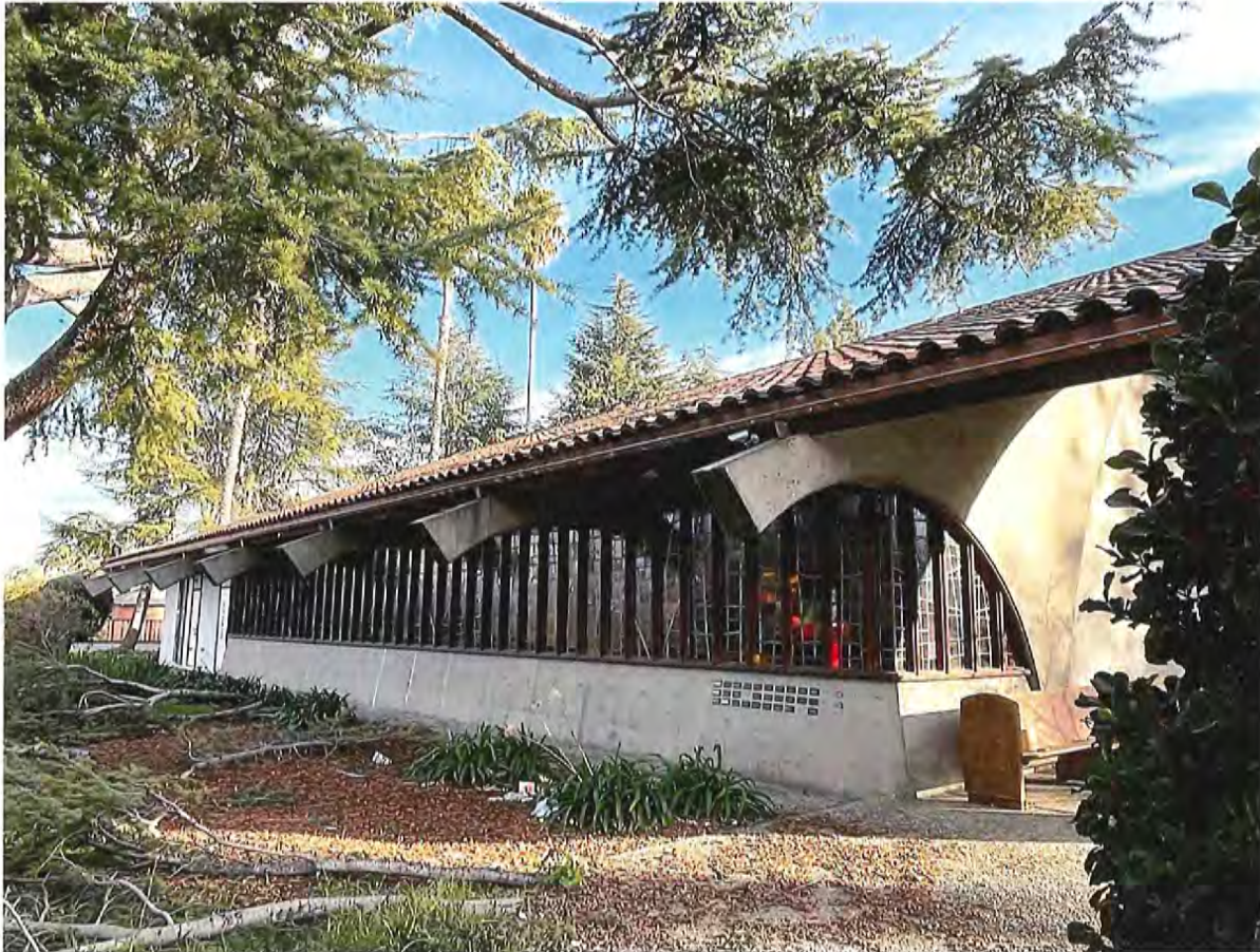
Photograph 3 1957 Pruneridge Avenue, Santa Clara View: North façade showing the heavy mullions in the windows and smooth stucco.
