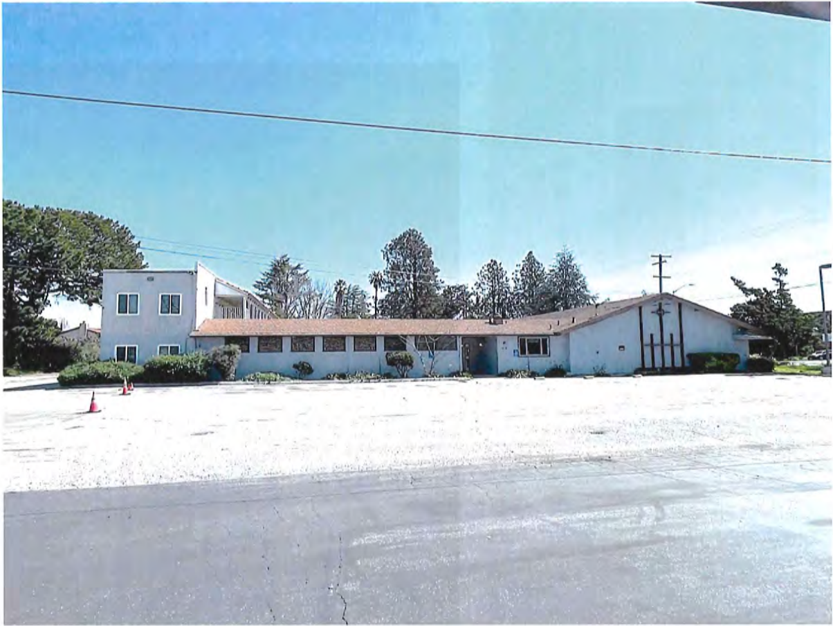
Photograph 11 1957 Pruneridge Avenue, Santa Clara View: Looking east at the rear of the classroom and parish hall complex.
