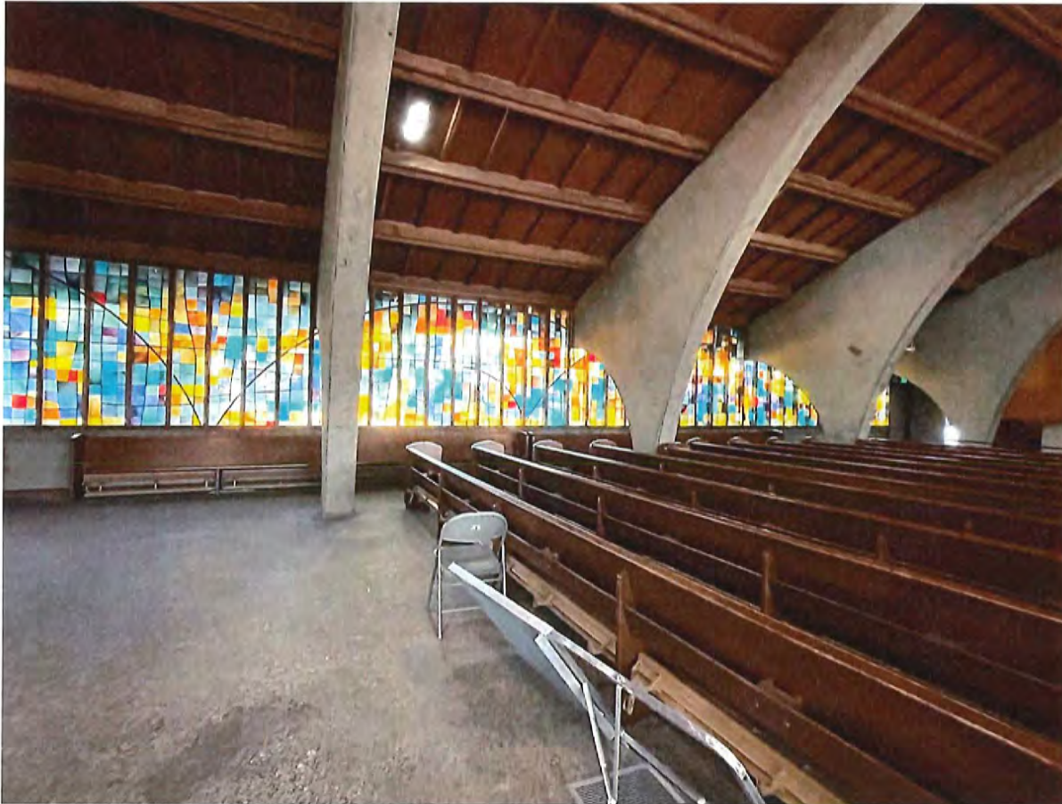
Photograph 9 View: Interior (north wall).
