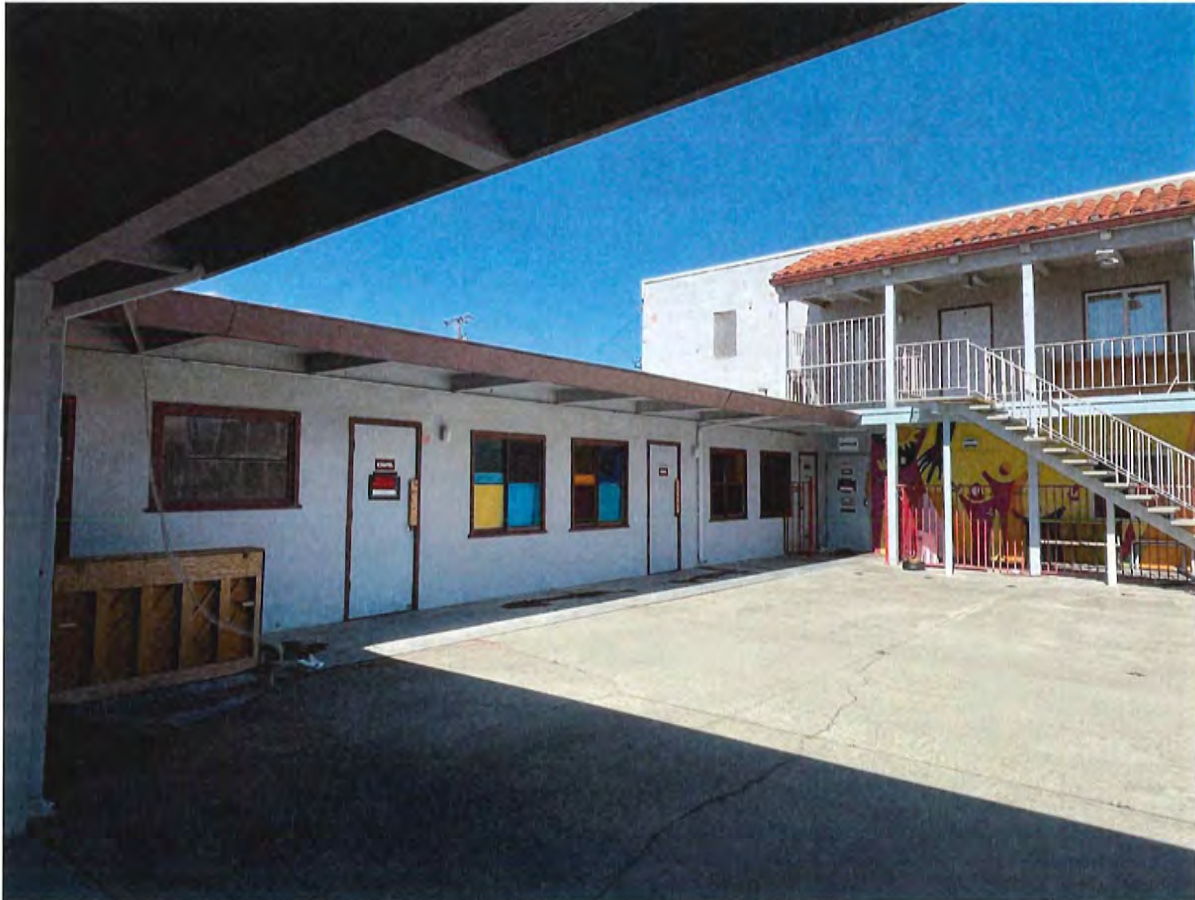
Photograph 12 1957 Pruneridge Avenue, Santa Clara View: Interior of courtyard showing the administration wing and two-story classroom building.
