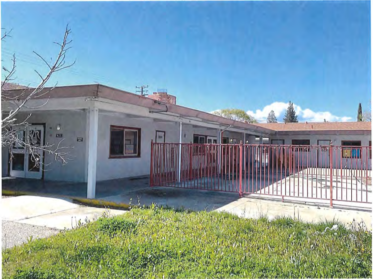
Photograph 15 1957 Pruneridge Avenue, Santa Clara View: Single-story admin building on the south side of the courtyard.
