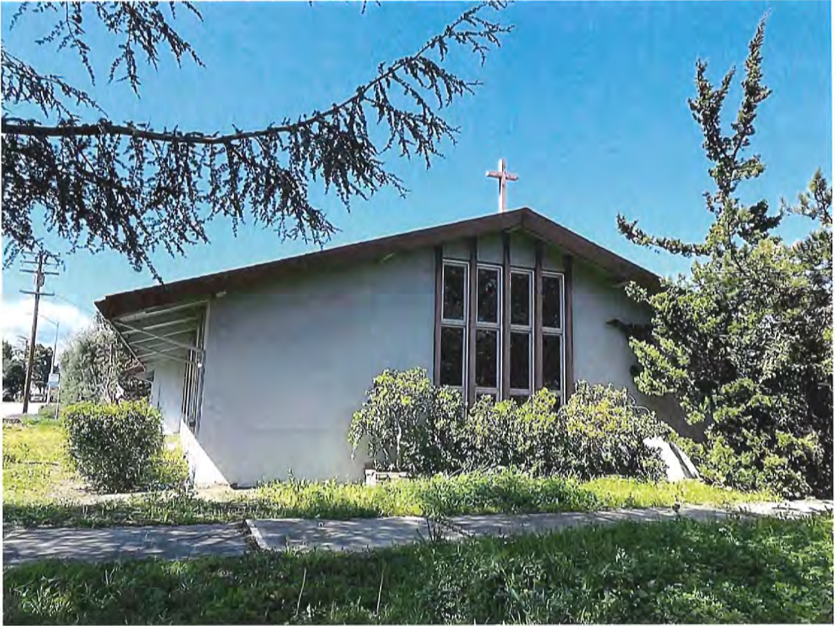
Photograph 17 1957 Pruneridge Avenue, Santa Clara View: East end of the Parish hall with broad overhanging eaves with angular downspouts on the south façade.
