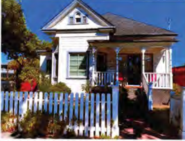
Photograph 5 1285 Jackson Street. View Front facade showing the steep steps to the first level of the house, approximately 4 feet above grade. This house shows the most remodeling and loss of architectural details yet retains a visual connection to the other two homes.
