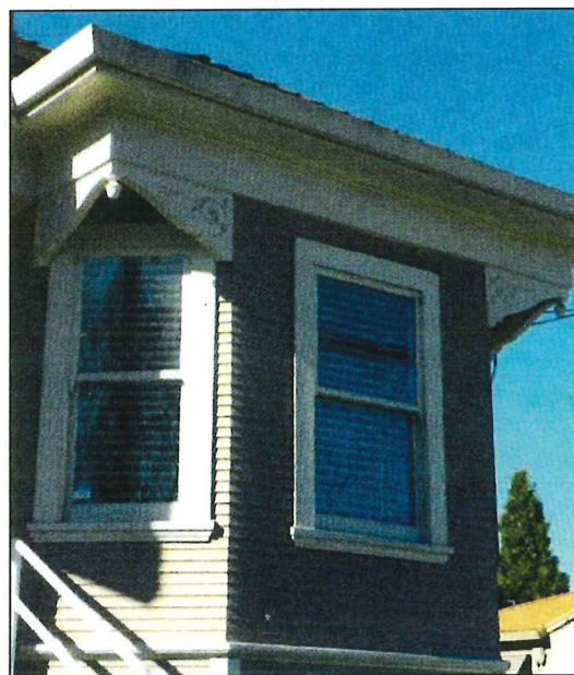
Photo No: 100_2399 View: Decorative bay window brackets and drop pendants Photo Date: January, 2019; Camera Facing: NW
