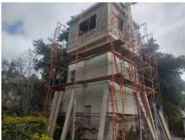
Repairs to Harris Lass
