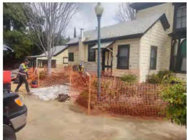
Repairs to Harris Lass
