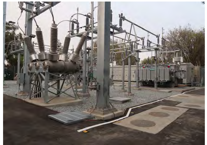
Serra Substation Rebuild
