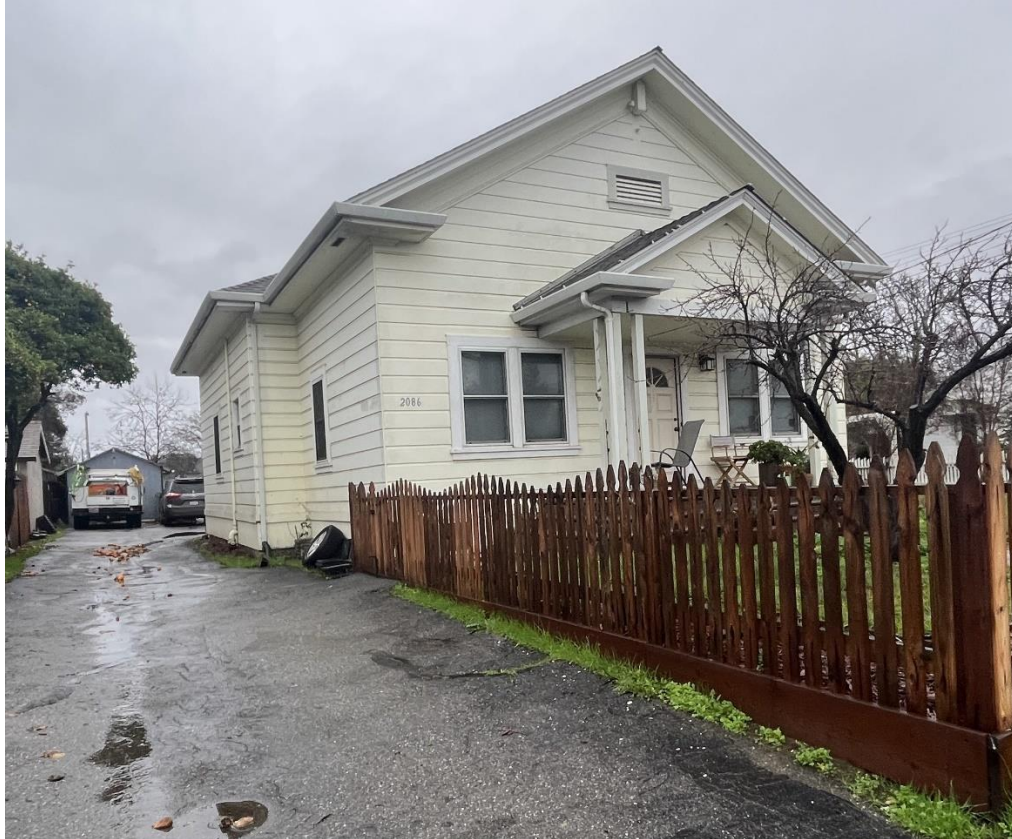
Figure 3. The building at 2086 Agnew Road, view of the north and east facades (Imagery date January 2023).
