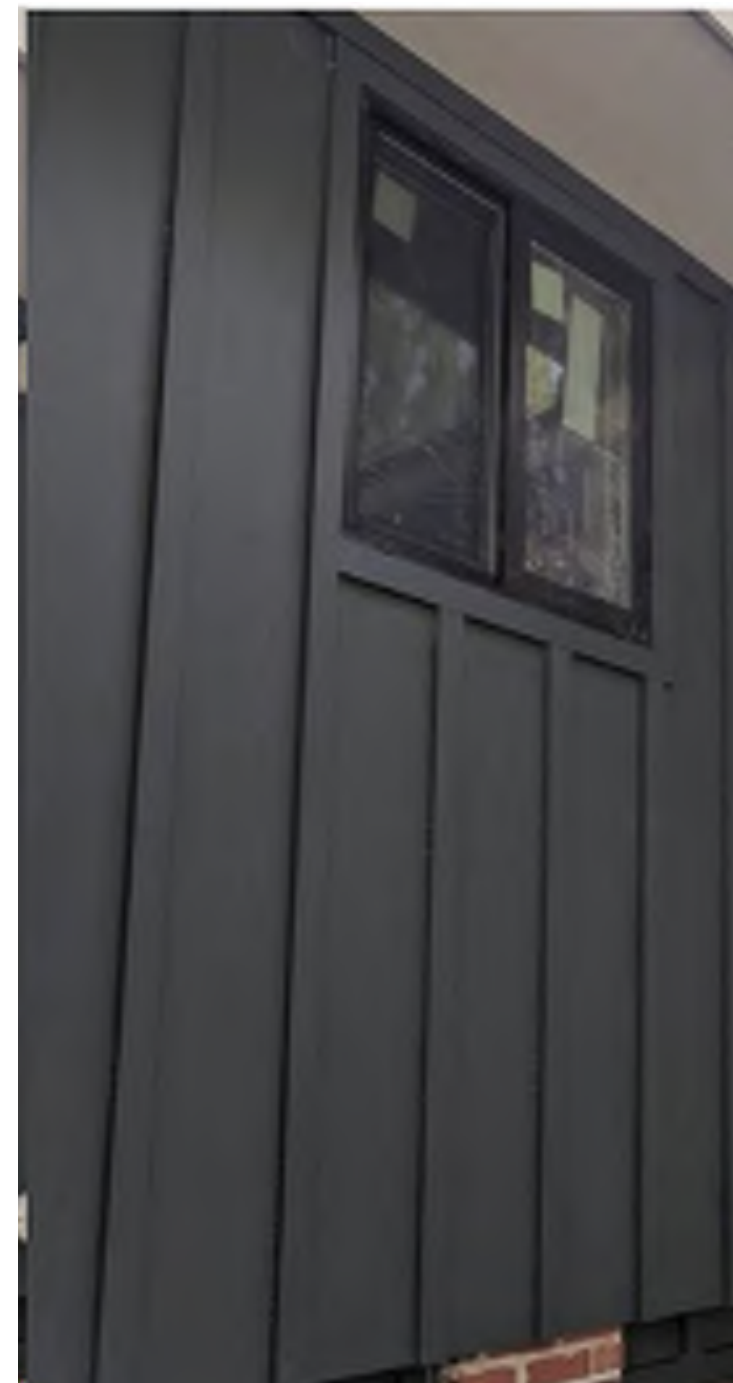
BOARD AND BATTEN SIDING - PAINTED LIGHT GREY
