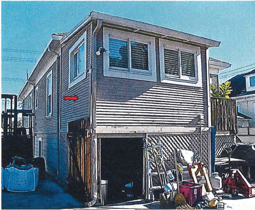
Photo 5. ➡ View of the existing, projecting “historic” sunroom with its narrow shiplap siding. The walls are proposed to be repaired and then reconstructed and incorporated into the new addition. The non-original windows will be altered.
