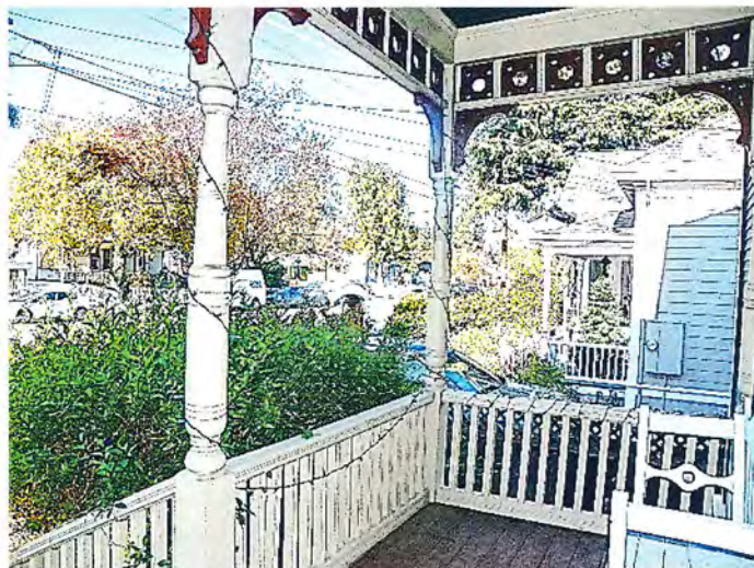
Photo No: 100_3320; View: Looking out through open end showing porch columns with brackets, frieze and balustrade. Photo Date: December, 2023; Camera Facing: WNW.
