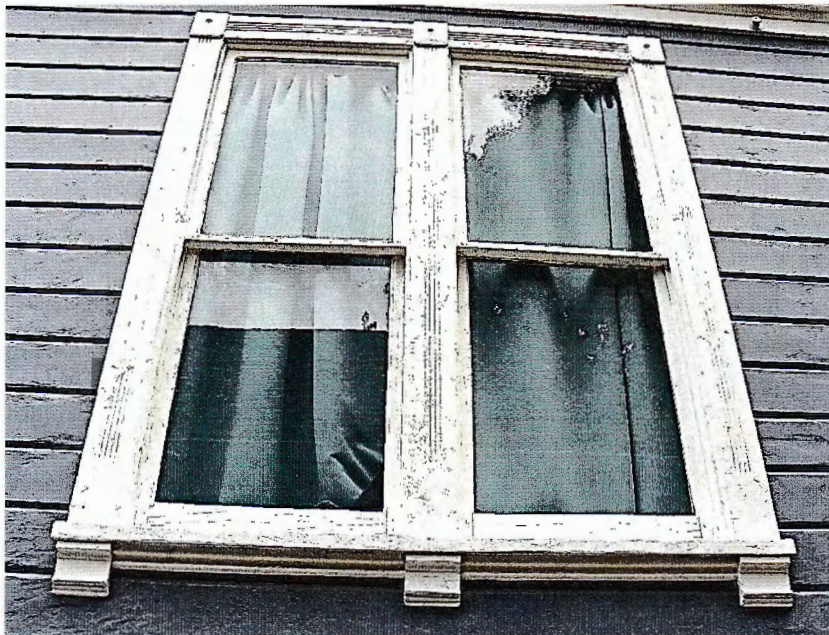
Photo No: 100_3670; View: Typical pair of dbl-hung windows with fluted trim & corner blocks and brackets under the projecting sill; Photo Date: 8/2/ 2024; Camera Facing: W.
