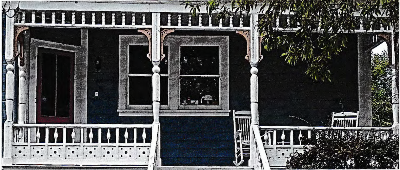
Photo No: 100_3643; View: Side Porch showing entry & ballustrade with Eastlake blocks; Photo Date: 8/2/2024; Camera Facing: SW.
