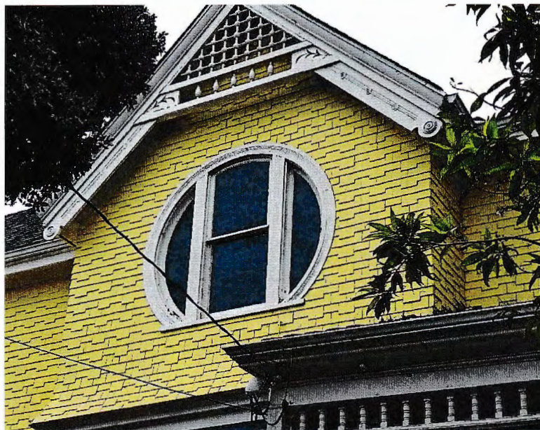
Photo No: 100_3640; View: E side-elevation Gable face with Moon window, Gable screen, carved bargeboards; Photo Date: 8/2/2024; View SW
