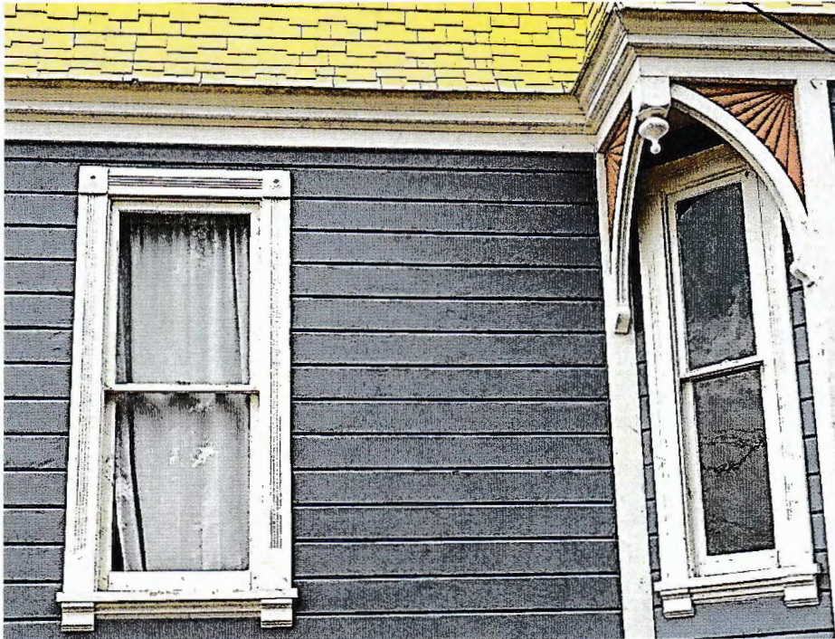
Photo No: 100_3647; View: Typical single dbl-hung window with fluted trim, corner blocks, brackets and cut-away bay window with sunburst brackets and drop pendant; Photo Date: 8/2/ 2024; Camera Facing: W.
