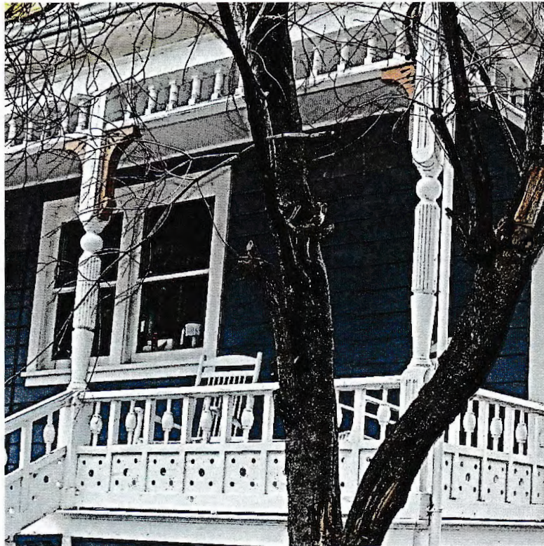
Photo No: 100_3648; View: Side Porch showing Eastlake block & rod and spindle ballustrade, fluted colonettes with brackets and turned post freize; Photo Date: 8/2/2024; Camera Facing: SW.
