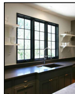
DET. 3 - MILGROD OR SIMILAR CASEMENT WINDOWS WITH BARS VINYL OR FIBERGLASS & DARK GREY COLOR
