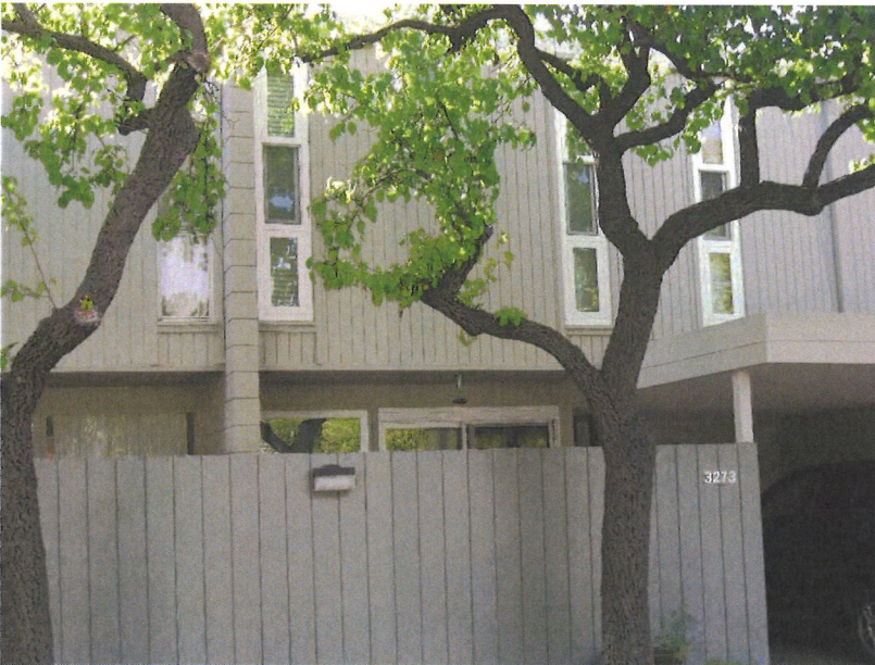
Photo 32 Building 14 east façade with original aluminum framed windows (left) and replacement vinyl framed windows (right), camera facing west
