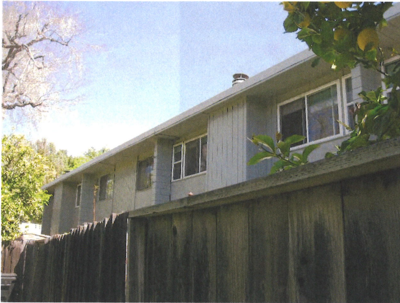
Photo 32 Building 14 east façade with original aluminum framed windows (left) and replacement vinyl framed windows (right), camera facing west
