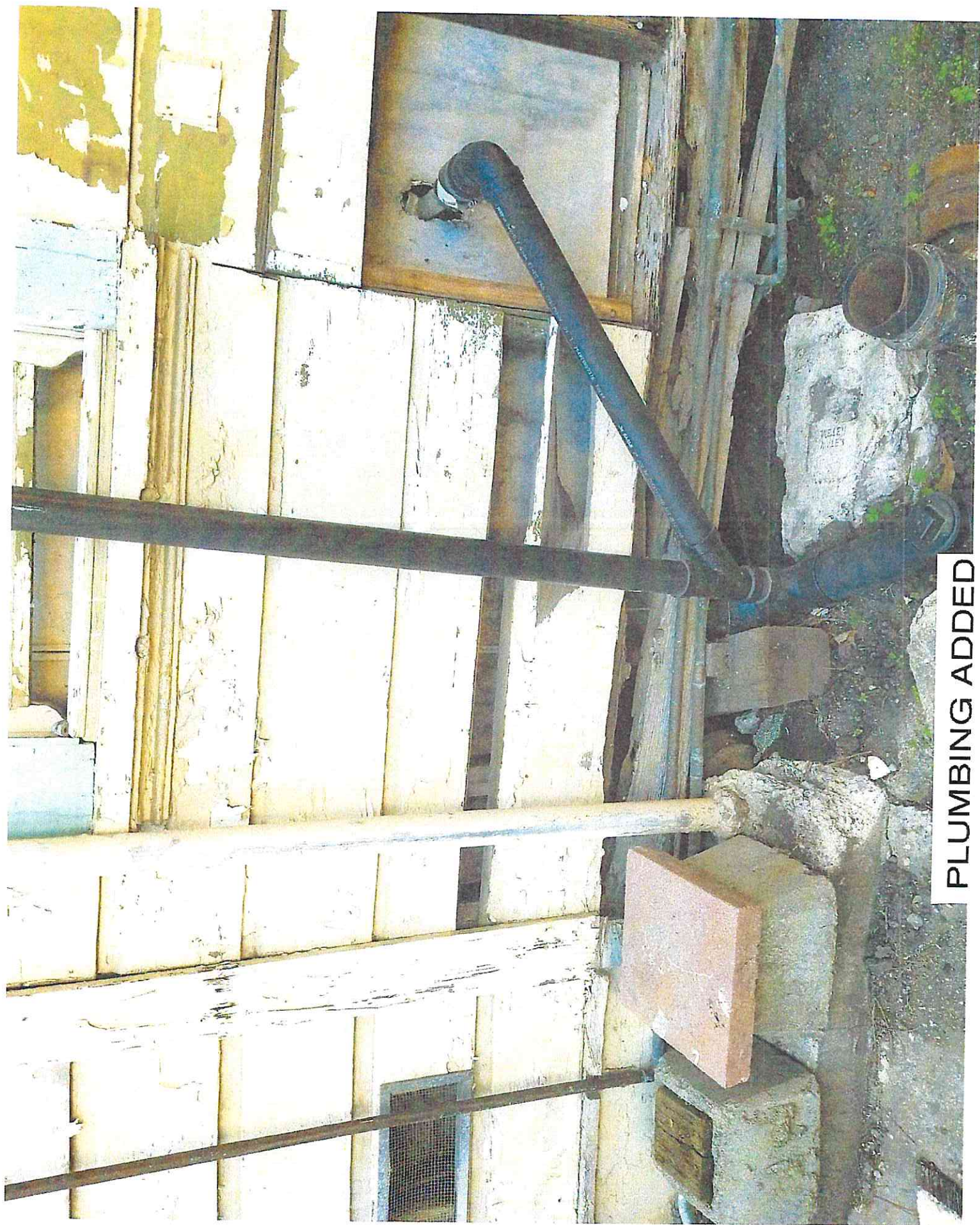
DETERIORATED FRAMING, SIDING AND FOUNDATION
