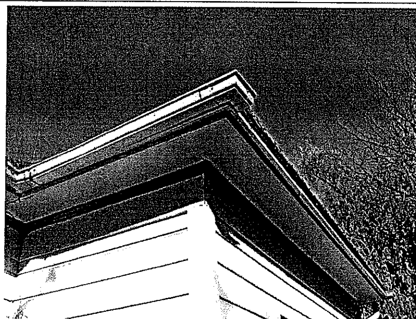
Photo 6: Detail of eaves showing deterioration.
