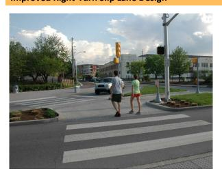
Right-Turn Slip-Lanes can be improved for pedestrian safety by shortening the turn radius to require vehicles to turn more slowly or removing slip lane entirely. Other improvements include refuge islands and marked pedestrian crossings that are perpendicular to the slip-lane (or as close to perpendicular as possible) so that people are clearly visible to oncoming vehicles.
