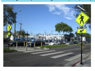
Rectangular Rapid-Flashing Beacons are useractivated pedestrian signals that use flashing yellow lights to alert motorists to the presence of pedestrians in the crosswalk. They can be installed in mid-block locations or at intersections where a full traffic signal is not warranted.
