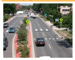
Advance Yield Lines are triangular pavement markings placed in advance of a marked pedestrian crossing to alert motorists to the upcoming crossing. From the advance position, motorist visibility of the crosswalk is also improved. Advance yield have been shown to increase yield rates. Stop lanes are placed in advance of a stop sign and alert motorists of where they should stop.
