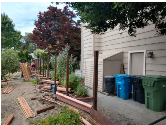
Morse Mansion Good Neighbor Fence Before
