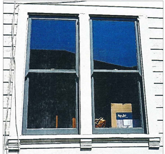
Photo No: 100_2661; View: Typical wooden windows with brackets, circa original 1893 construction; Photo Date: August, 2020; Camera Facing: NW.
