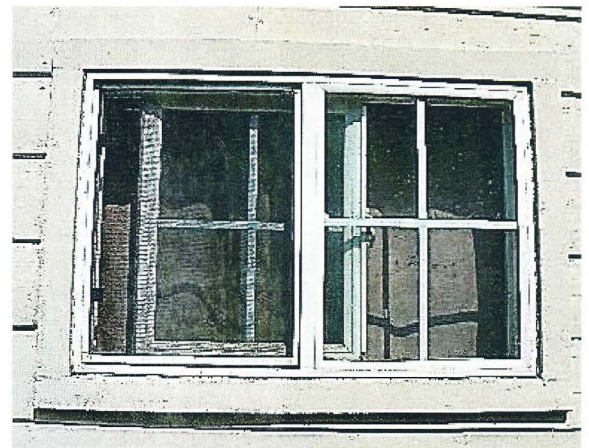
Photo No: 100_2660; View: Typical vinyl-clad sliding windows in S side-elevation rear extension. Photo Date: August, 2020; Camera Facing: NW.
