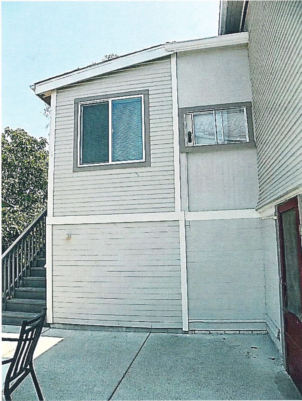
Photo 2. View of the rear two-story projection's (west) side elevation. Note the two existing non-original sliding windows in the projection's main/living level. A new 2'8" x 6'8" French door and a 4' x 6'8" glass sliding patio door are proposed to be placed in the solid basement level's wall beneath these windows.
