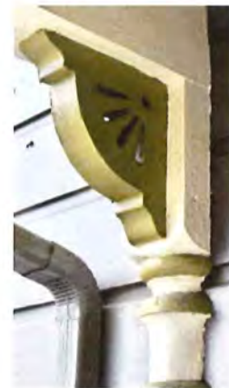
Front porch, turned porch post, and incised brackets
