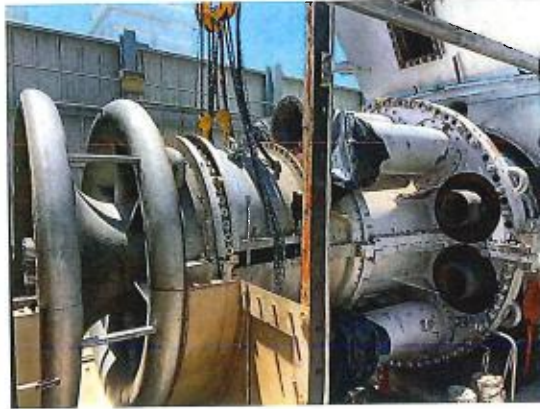
Compressor Inlet / Combustion Can Disassembly
