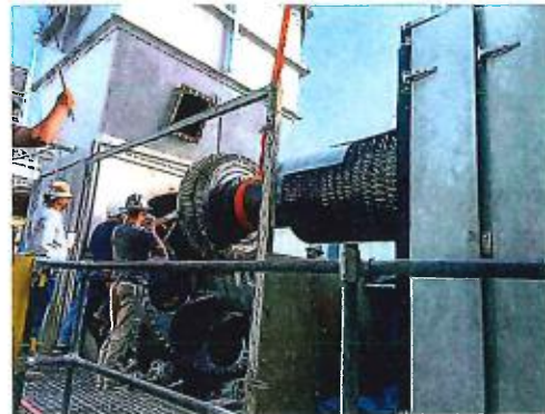
Unit 1 Rotor Installation
