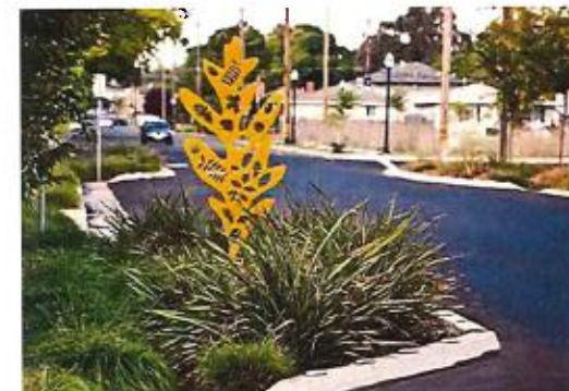
5.2.3.8C - Stormwater Planters in Parking Bulbout
