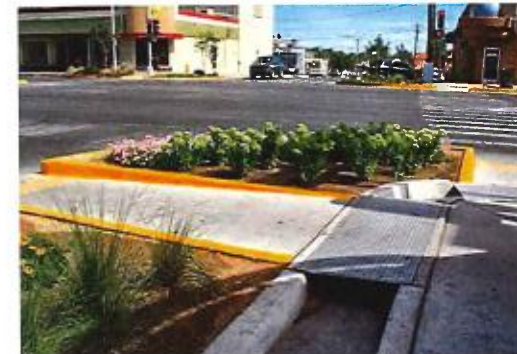
5.2.2.2 - Directional Ramps with ADA Access
