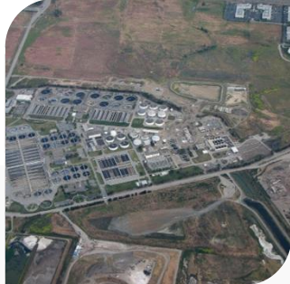
Regional Wastewater Facility
