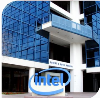
Major Data Center for Silicon Valley
