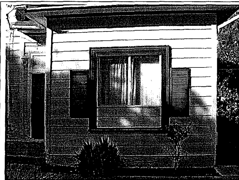
Photo 7: Detail of windows resized and replace with vinyl.
