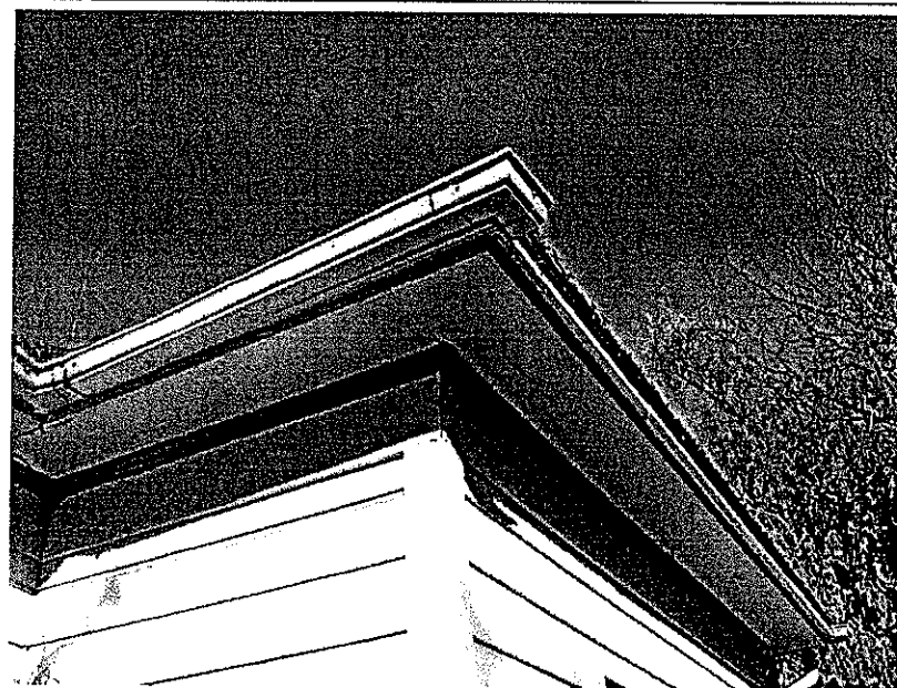
Photo 6: Detail of eaves showing deterioration.
