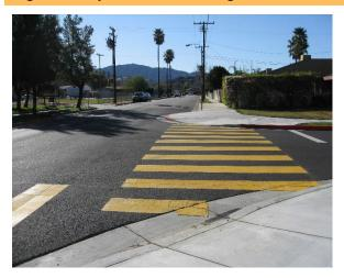
High Visibility Crosswalks are enhanced crosswalks that clearly define the pedestrian space and help to deter vehicle encroachment. The continental type shown here is one of the most common configurations.
