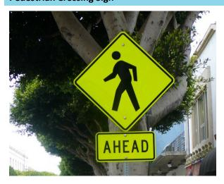
Pedestrian crossing signs alert motorists to the presence of a marked crosswalk. They can be placed parallel to or in advance of a crosswalk, and are particularly useful in locations where a crosswalk may not be expected by motorists.
