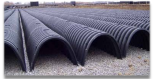
Figure 2-5 Subsurface infiltration system (Source: Conteches.com)
