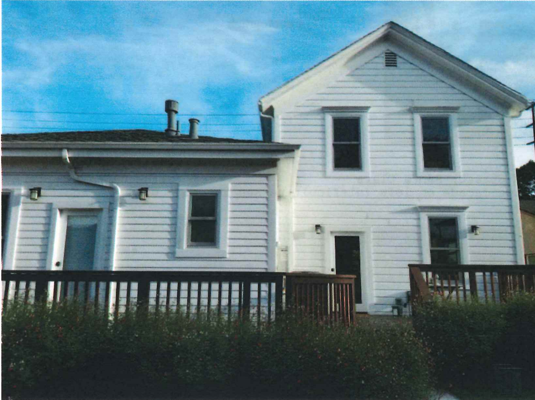
1217 Harrison Street, Santa Clara View: Rear façade, older addition on the left. Original house on the right. The rehabilitation retained the windows and frames, and siding. No new windows were added during the rehabilitation. Date: September 27, 2018
