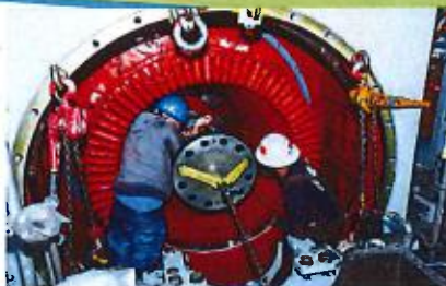
Steam Turbine Generator Rotor Removal
