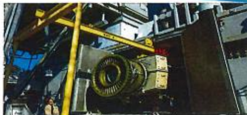
Gas Turbine Engine Removal
