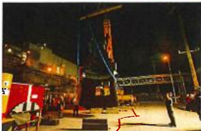
Steam Turbine Casing Flip
