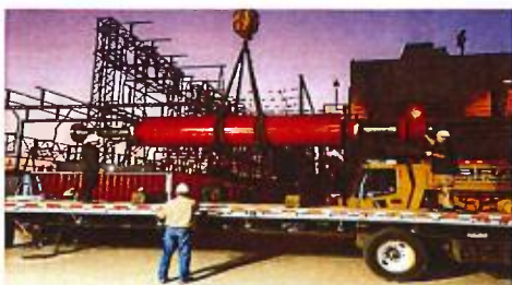
Steam Turbine Generator Rotor Trucking
