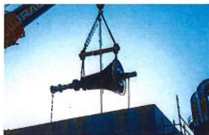
Steam Turbine Rotor
