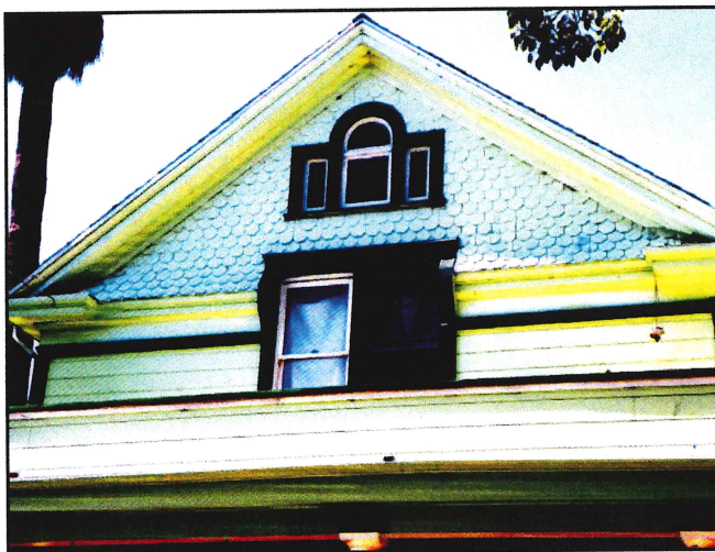
Photo No: 100_1889 View: Front facade gable detail showing Palladian window and fishscale shingles on gable face Photo Date: May, 2016 Camera Facing: NW
