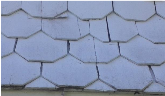
Figure 3 Fish scale shingles in need of repair
