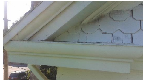
Figure 6 New section of cedar moulding, custom made to match existing pattern.
