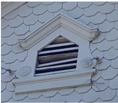
Figure 5 Louvered attic vent on rear gable
