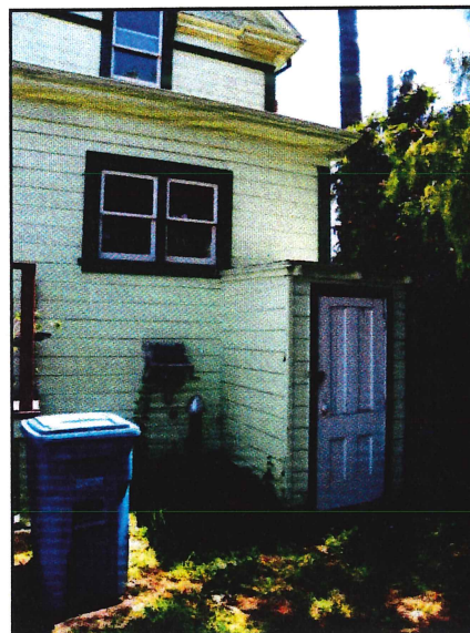
Photo No: 100_1899 View: Rear facade showing basement entry projection & replaced widows (2005) in rear porch Photo Date: May, 2016 Camera Facing: S
