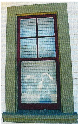
Photo No: 100_2541 View: Horizontally orientated, 4-over-1 double-hung window Photo Date: July, 2020 Camera Facing: WSW
