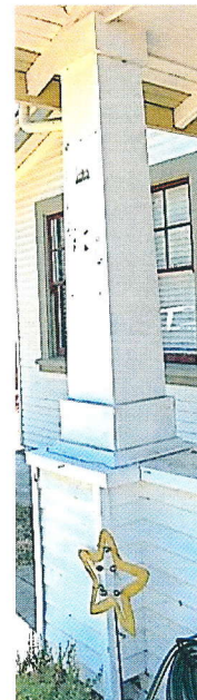
Photo No: 100_2551 View: sloping (battered) column on squared pier (exterior view) Photo Date: July, 2020; Camera Facing: SW
