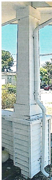
Photo No: 100_2587 View: sloping (battered) column on squared pier (interior view) Photo Date: July, 2020; Camera Facing: NE
