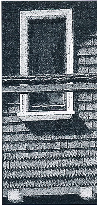
Gable detail showing decorative band of 4 rows of saw tooth shingles and two of the attic-story supporting squared brackets
