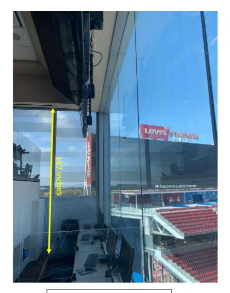
Image above represents the highest point Above Finished Floor (AFF) for all nine (9) windows. This information is provided for informational purposes only to assist the Contractor plan their installation.
