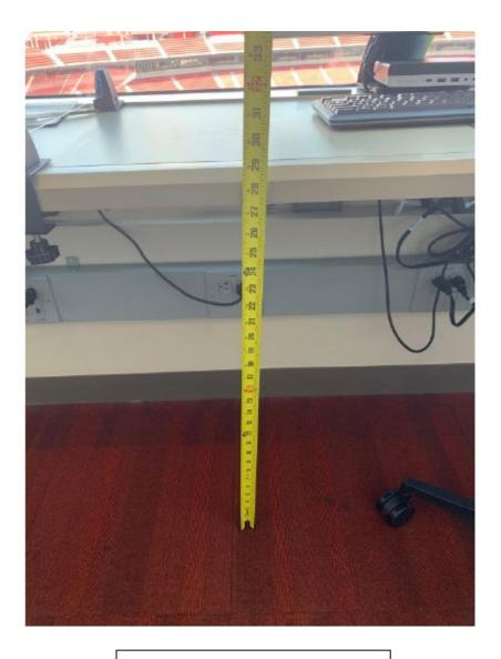
Image above represents the lowest point Above Finished Floor (AFF) for all nine (9) windows. This information is provided for informational purposes only to assist the Contractor plan their installation.
