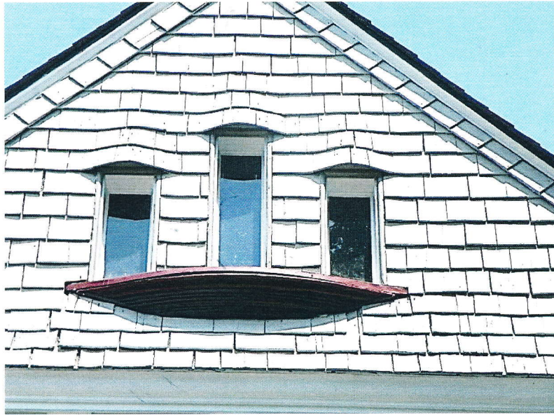
Photo No: 100_2746; View: Gable face shingle sheathing and windows Photo Date: August 2021; Camera Facing: NNW
